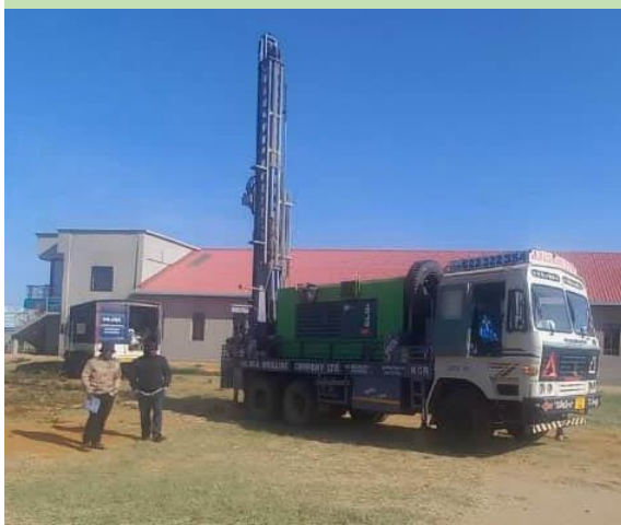
Drilling work in front of the new LEA boys' dormitory
